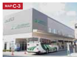
●JR Takayama Station Bus Terminal
